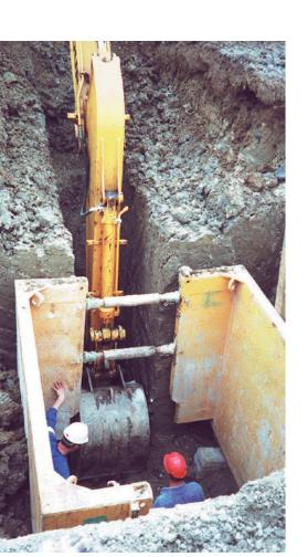
The Manhole Box is used when, in continuous pipeline trenches, wider areas for manholes need to be created. The plate body is U-shaped, and forms a recess of 0.40 m at each side of the trench. The result is a working area of up to 0.80 m wide.
